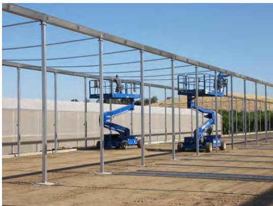
Early construction note the original screenhouse in the back
