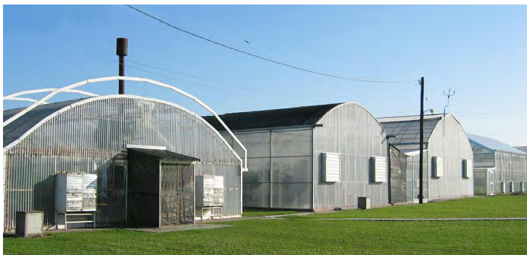
Fig. 1. Greenhouse facilities for biological indexing of citrus pathogens at the Estación Experimental Agroindustrial Obispo Colombres of Tucumán (EEAOC).
